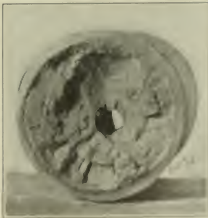
FIG. 2. SECTION OF 4-INCH EXHAUST PIPE SHOWING DEPOSITION
